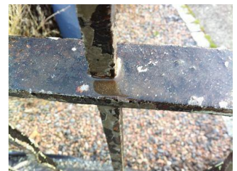
^ Saturate with Owatrol. Wipe off any excess to avoid 'skinning'
