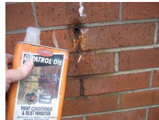
^ Broken anchor bolt rust stopped with Owatrol
